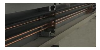
f.) Alternative piping method 2: QLCI units can allow the piping runs to be in the front of the units above the hydronic coil. This allows the QLCI to be mounted to the 2x4's first, then connect the ductwork before making the piping connections. The feeding pipework can be routed through the side wall knockouts. QLCI's and piping connections can be connected in the front as shown below.
