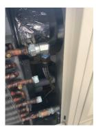
b.) The vertical chilled/hot water pipes are connected via flexible hoses run through a pipe work knockout on the top or side of the unit.
