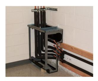
b.) Install threaded  $\frac{1}{2}$  NPT connections (provided by others) on each pipe or solder straight end connections 2" to 3" from the point where the QLCI units connect to each other along the wall as shown below.
