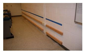
b.) The **2x4 Mounting Boards** should run the length of the QLCI installation (not individual units). The **2x4 Mounting Boards** should stop 1.5" from edge of wall to allow end unit side panel to set flush against the wall.
